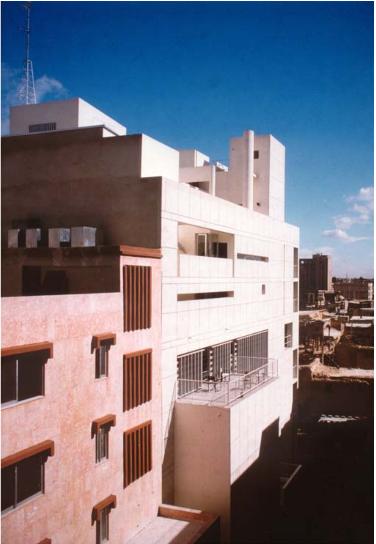
View of South Elevation and adjacent Building
