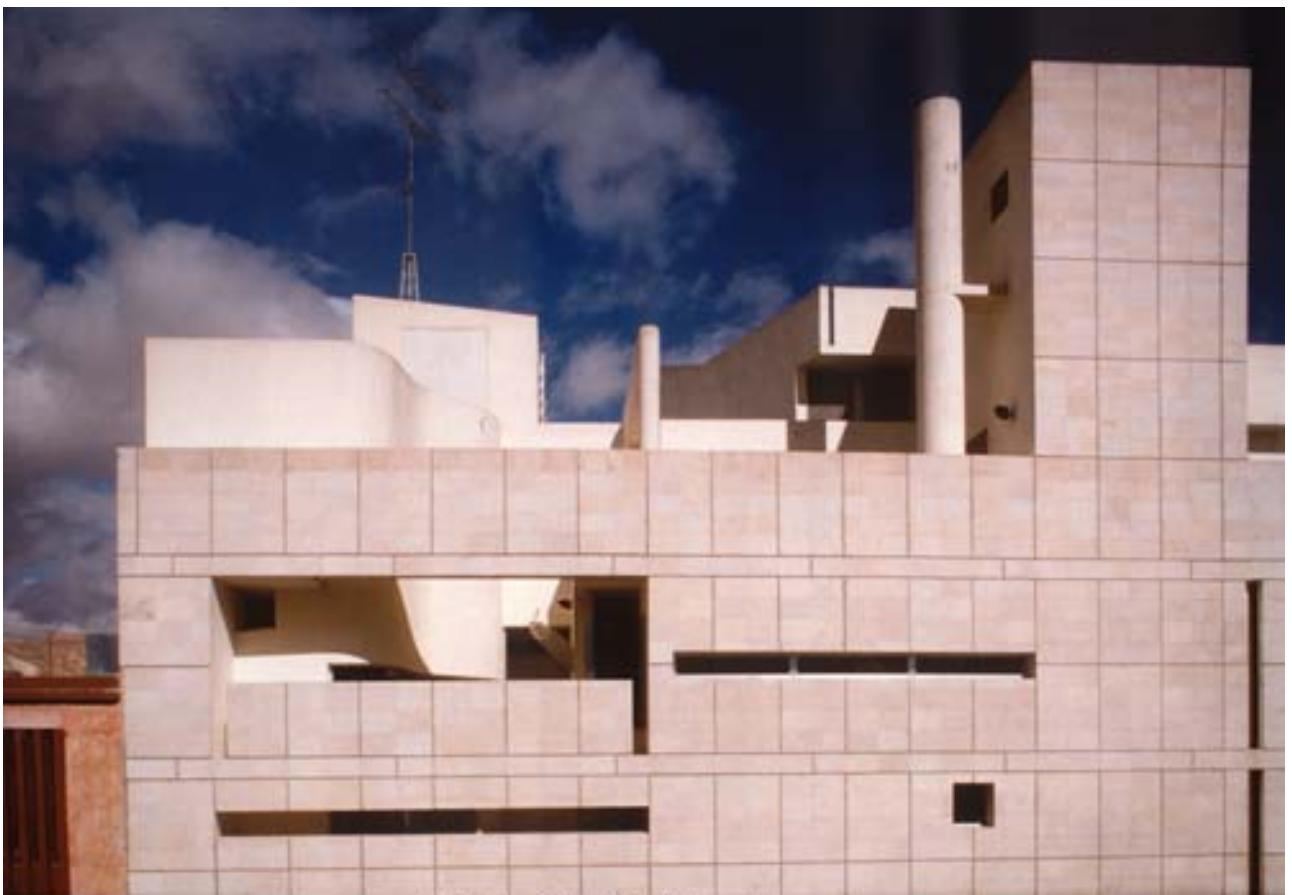
Detail of the Southern Façade
