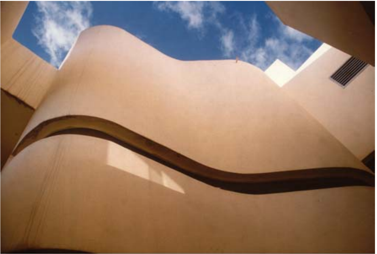
Detail of the Southern Façade
