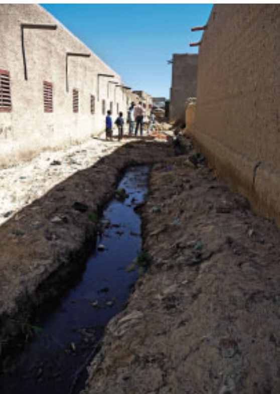
Open sewers and poor drainage were serious health hazards in Komoguel.
