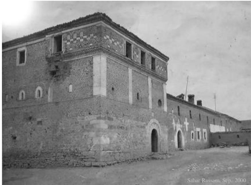
Figure 1: kulla of M. Gega, Gjurrakoc, Istog, as it used to be with the attached annex. Constructed of stone and brick. Taken from an old picture.
