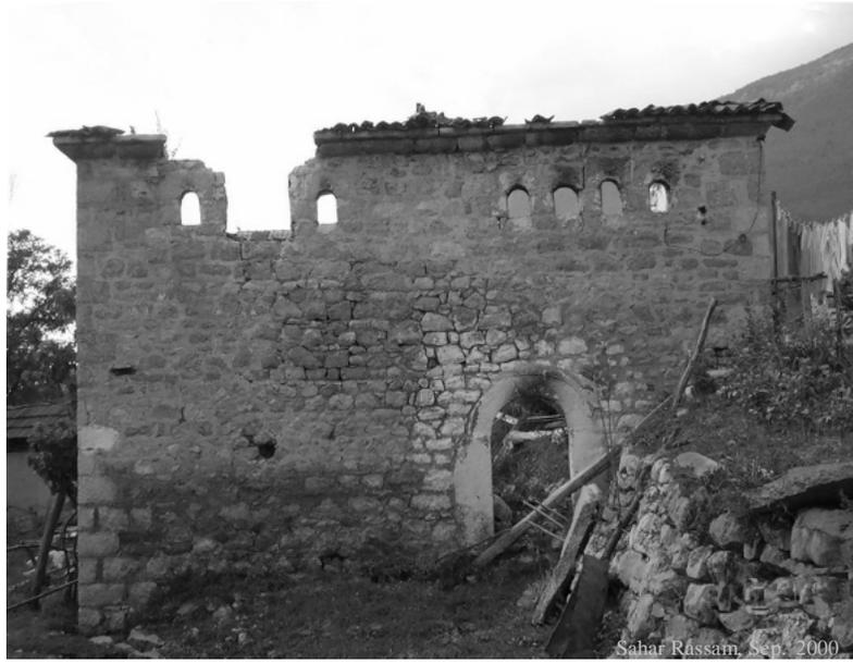
Figure 2: Kulla of R. M. Avdijaj, Syne, Istog, constructed of stone.
