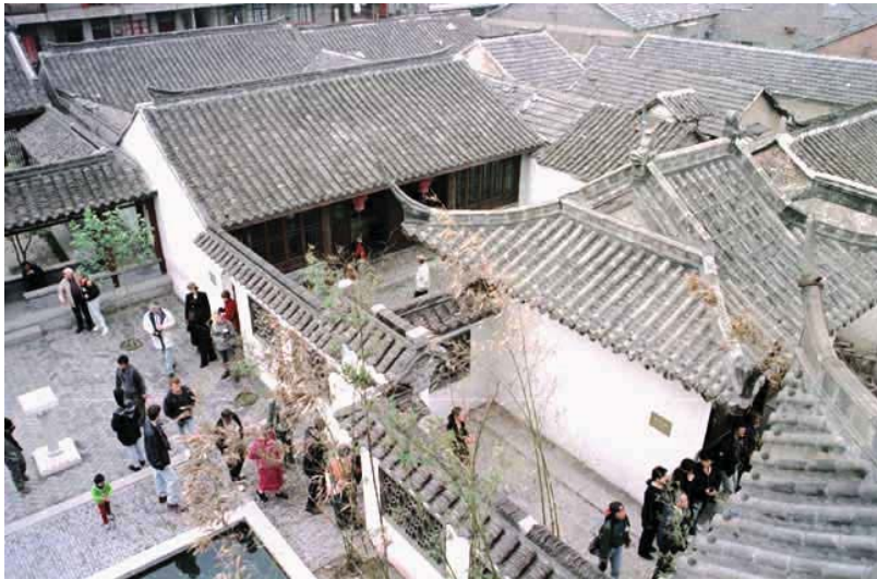
Figure 4: Traditional residential buildings in Gao-you, Jiang-su Province have offered high density living comparable with modern-day expectations but better suited to Chinese life-styles and social fabric (Source: Author).
