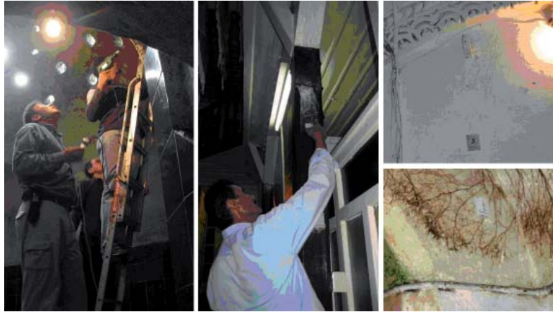
Figure 1: Installation of Internal Data Loggers in Hammāms of Cairo (left), Ankara (middle), and Fez (right). (Source: Authors).
