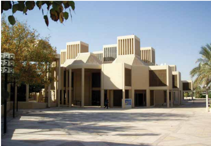
Figure 2: The Use of Repetitive Pre-cast Elements for Both Cladding and Structural Walls, A Major Design Feature that Characterizes the Design of All Educational Buildings. (Source: Author).
