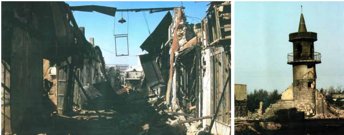
Figure 3: Damaged traditional buildings. Left: Old market – Right: Old mosque minaret. (Source: Y. Mahgoub).
