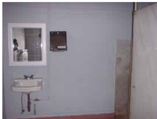
Outdated restroom facilities.
