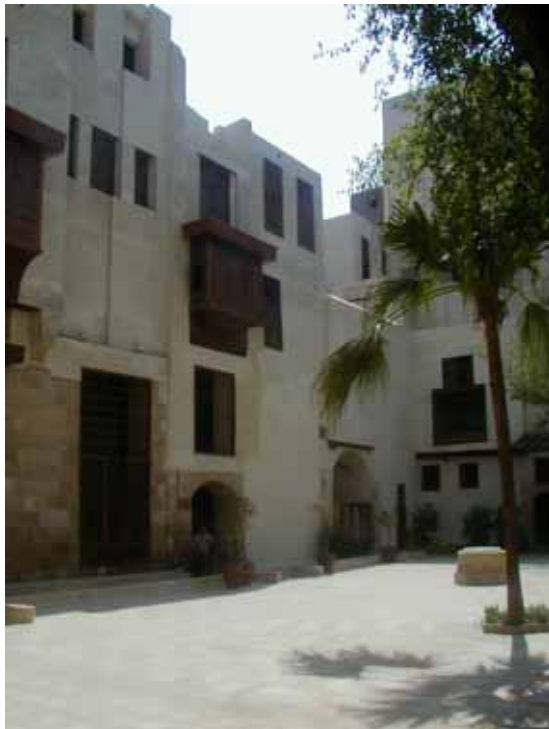
A. Figure 11-A: The Back Yard of Al Suhaymi House After Restoration.
