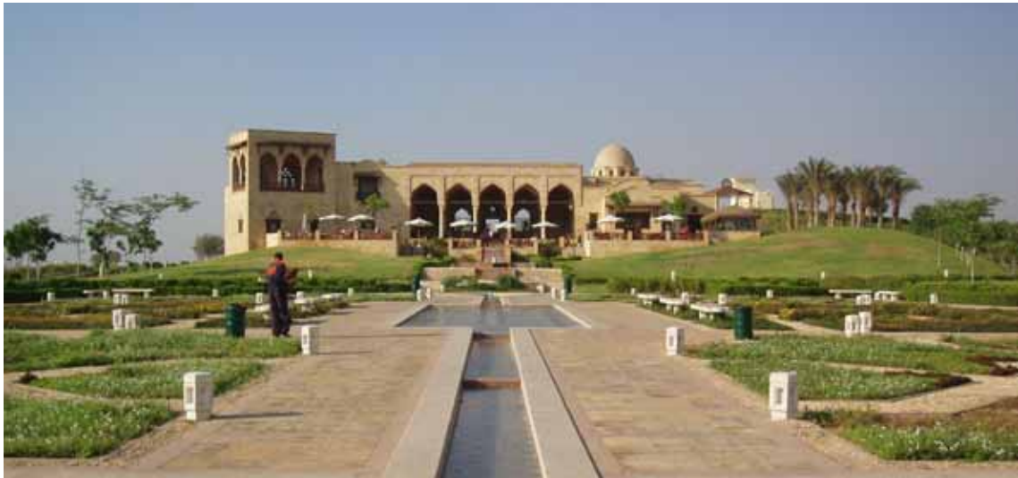
B. Figure 12: Al Azhar Park; A new Lung for Cairo's Urban Core
