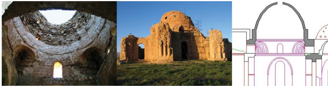
Figure 3: Domes of Sarvestan palace with primary samples of squinches, Sassanid era. (Sources, photos: www.treearth.com/gallery/Middle_East/Iran/East/Fars/Sarvestan/ ; The vertical section: Authors).
