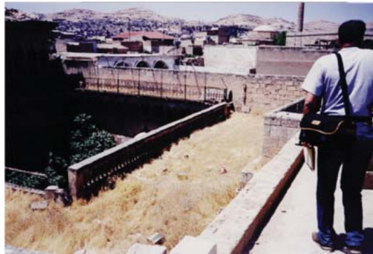
Figure 15: Roof garden (Source: Authors).
